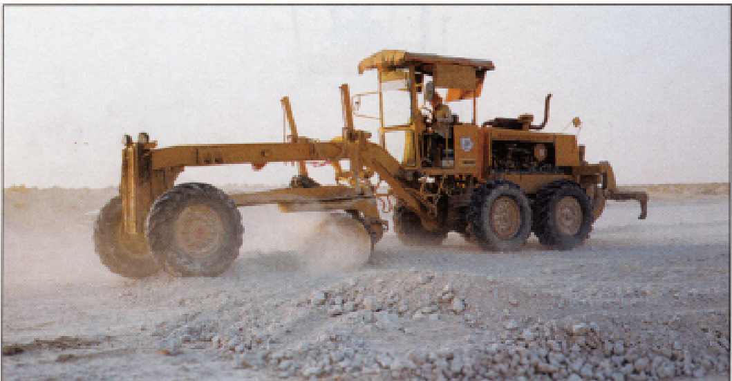
Grader spreads marl at a life support area.
