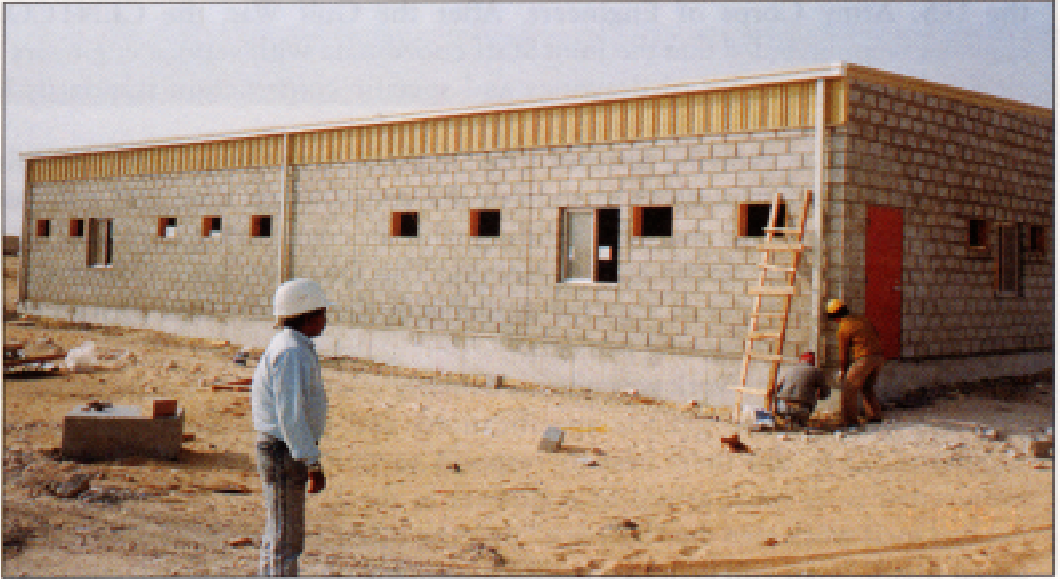
Cement masonry building under construction at a life support area.
