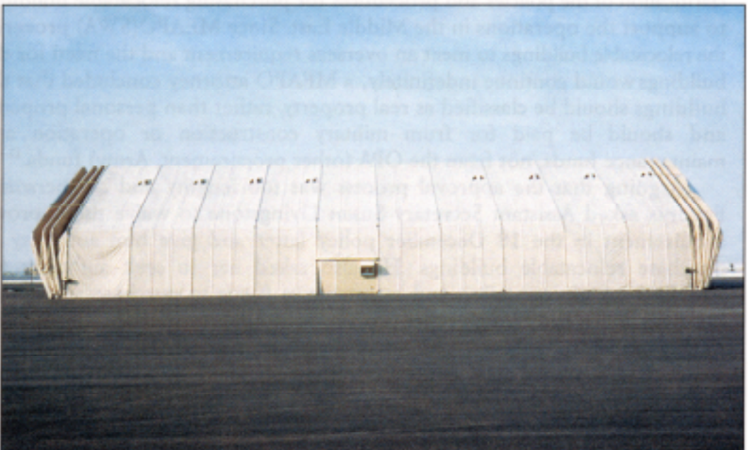
Side view of a clamshell building at King Fahd International Airport. The ends of the clamshell are opened and closed by either a band-cranked or a generator-driven winch.
