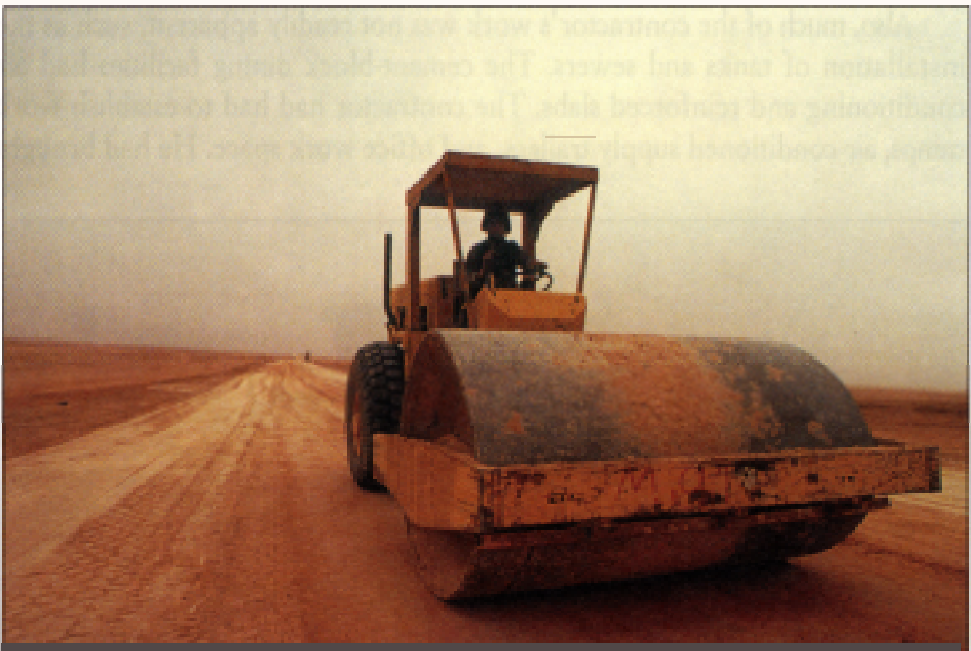
Soldiers from the 20th Engineer Brigade compact the ground for a new road in Southwest Asia.
